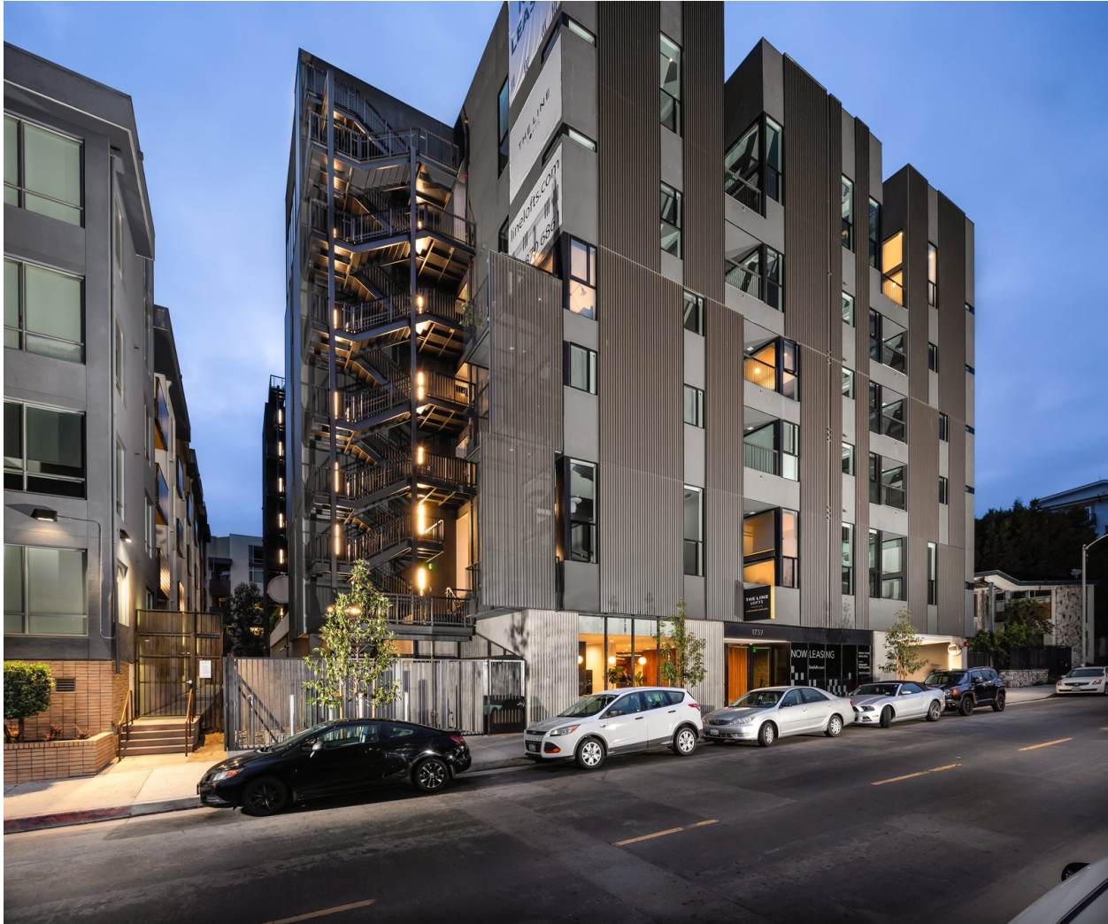
The distinctly modern exterior of The Line Lofts.
